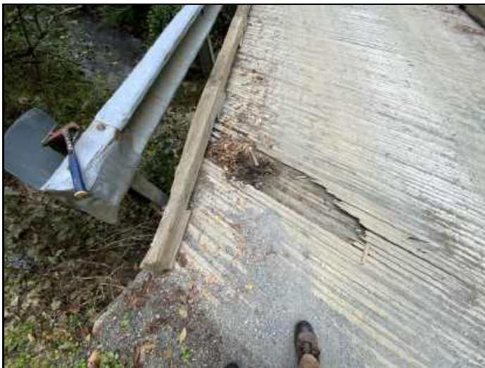
Abutment 2 downstream end of deck
