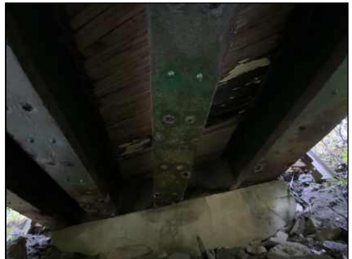
Deck over abutment 2
