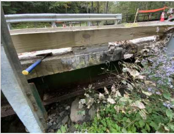
Abutment 2 downstream end of deck
