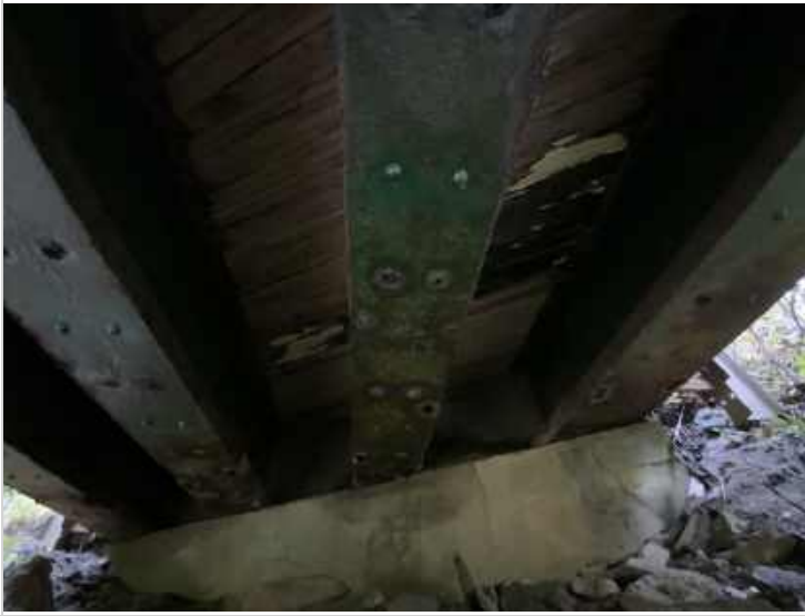
Deck over abutment 2
